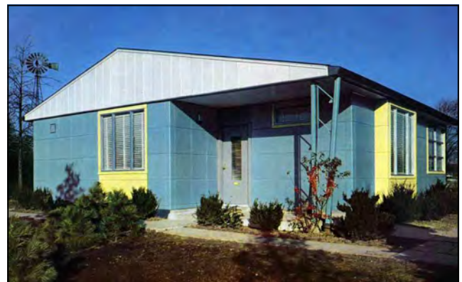
The New York State Lustron Project documented 70 pre-fab, all-steel ranch houses from the 1950s. The survey resulted in several National Register listings in a number of New York State communities.
