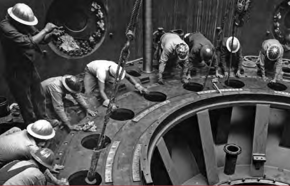
Turbine Construction, Moses-Saunders Power Dam, 1957. Courtesy New York Power Authority.
