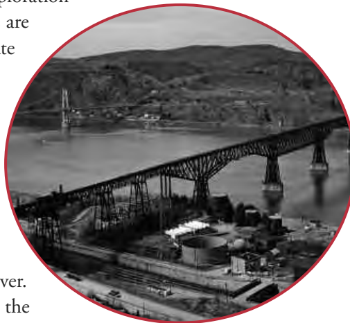
Aerial view of the Poughkeepsie Railroad Bridge, 1978. Courtesy Historic American Engineering Record.
