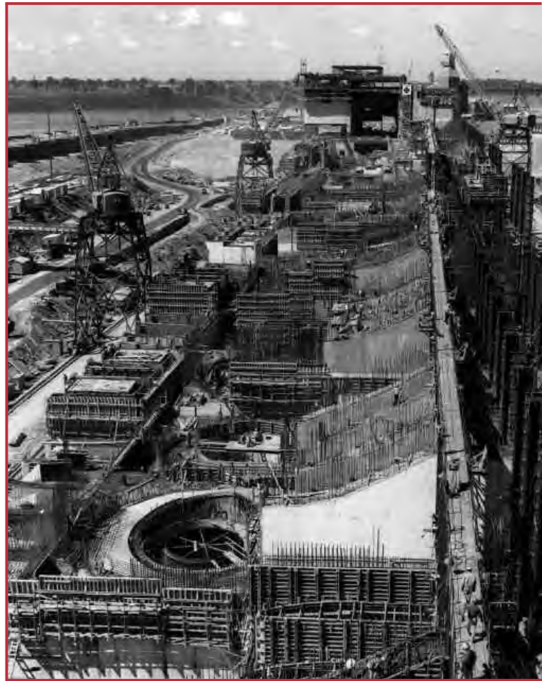
Moses-Saunders Power Dam Construction, 1957. Courtesy New York Power Authority.
