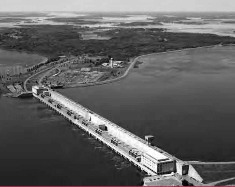
Moses-Saunders Power Dam, undated. Courtesy New York Power Authority.
