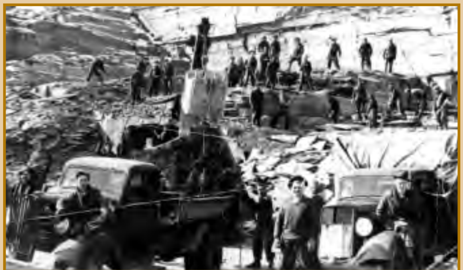
CCC workers excavating stone at a quarry in Montour Falls for Watkins Glen State Park, courtesy Schuyler County Historical Society.
